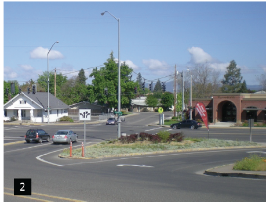
The above photos show Freeman Road as it approaches East Pine Street from the south. [1] a stop ahead sign is used to warn drivers where a vertical drop limits visibility [2] once down the hill, a horizontal curve to the right can make visibility difficult as well
