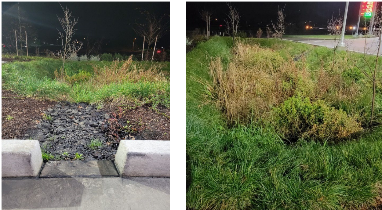
Figure 4.1. An established Rain Garden on a commercial lot, view from an inlet (left), and looking into the facility inlet (right).
