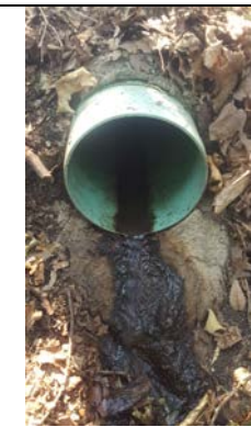
Coleman Ck. outfall 5
