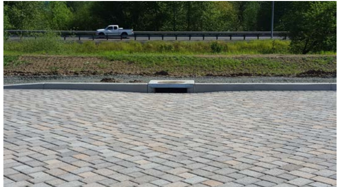
Permeable paver parking lot in City of Phoenix downtown redevelopment.
