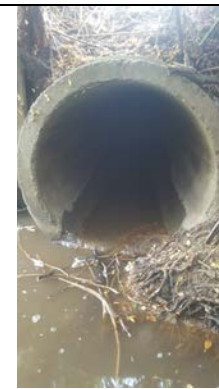
Payne Ck. outfall 5
