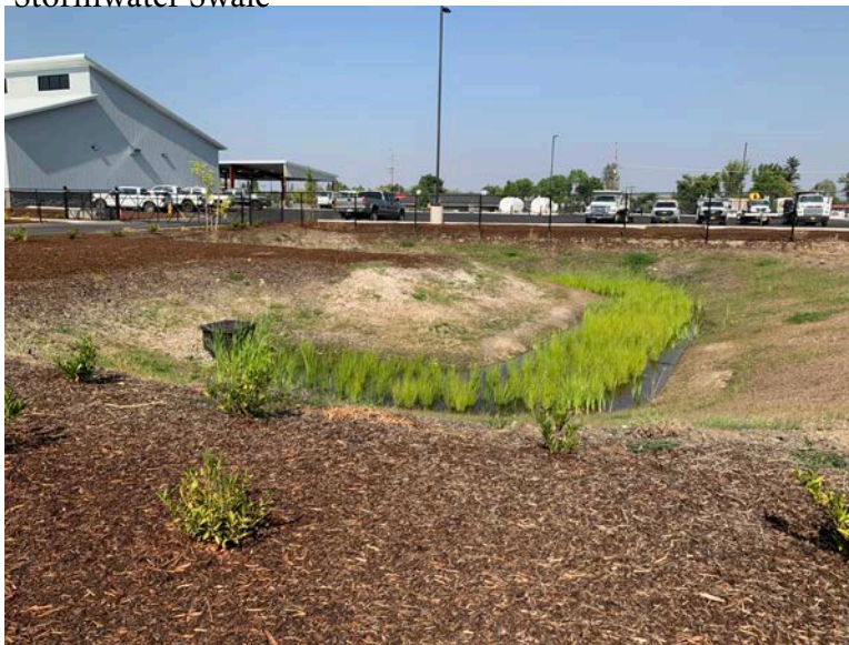
Stormwater Swale
