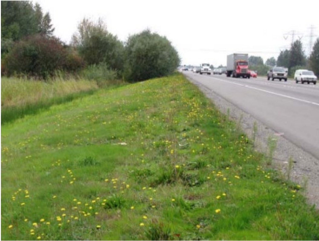
Figure 3.4. A vegetated Filter Strip runs along the left side of this path.
