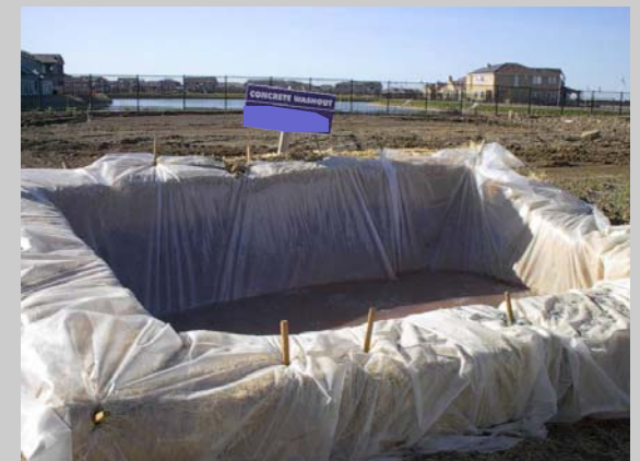
An example of a properly designed concrete washout. Washouts can be scaled down for use on smaller projects.
