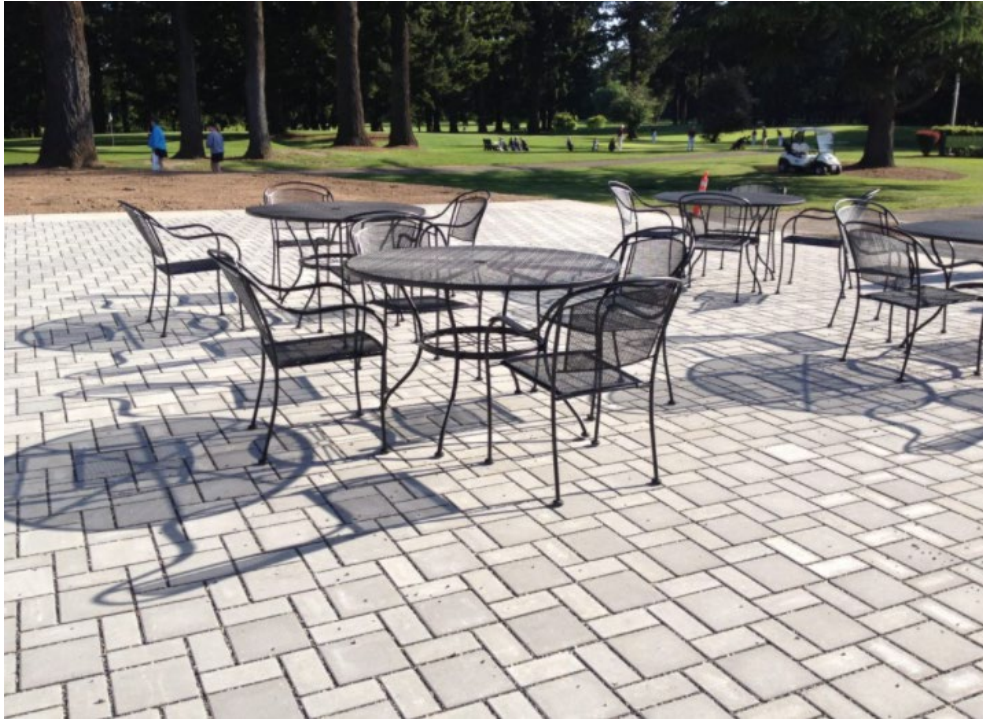
Figure 3.3. Pervious surface not intended for vehicular use.
