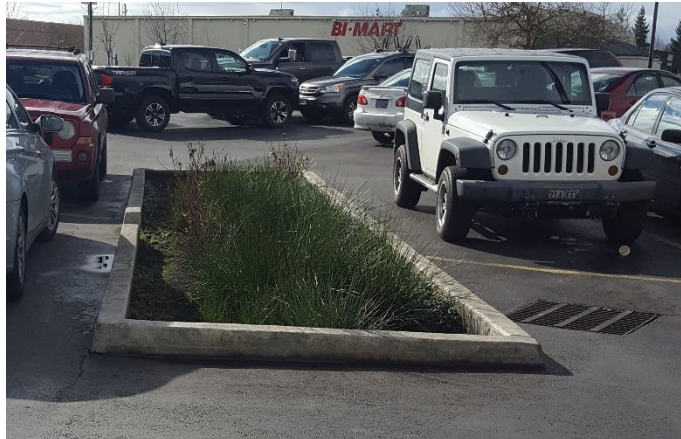
Figure 3.2 Stormwater Planter.
