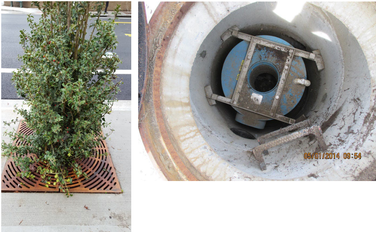
Figure 4.11. Filterra Units (left) and Filter Cartridge Units (right) are examples of proprietary Treatment devices that meet the requirements of this Design Manual.
