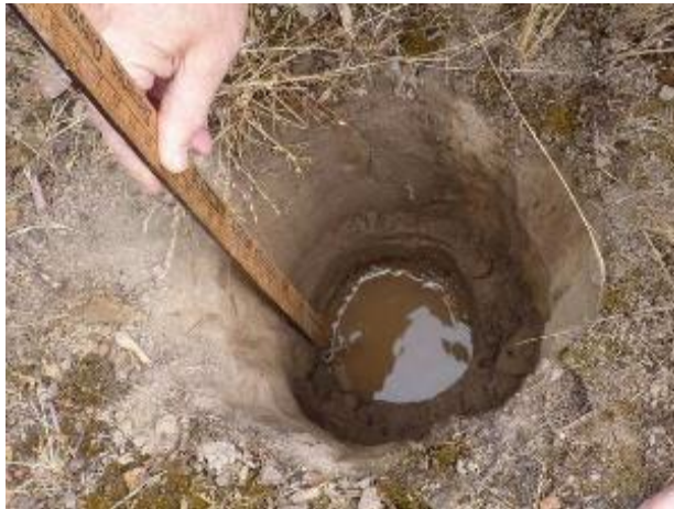
Figure A-2. A shovel was used to dig most of the way then a 6" diameter post hole digger was used to reach the proposed bottom elevation of a rain garden. Measure the drop in water from a known, stable marker.
