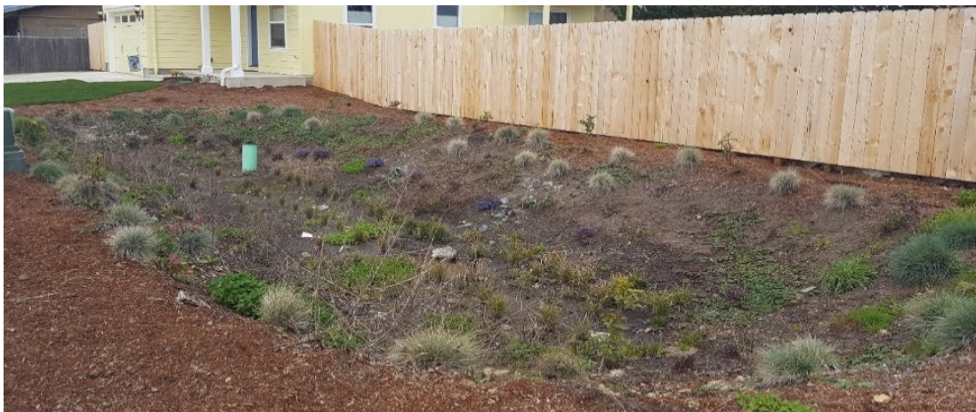
Figure 3.1. Rain garden six months after planting.
