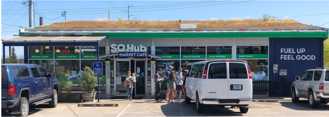
Figure 4-12. Vegetated Roof example on a convenience store.
