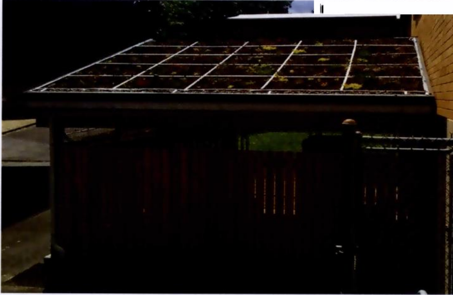
Figure 4.1. Growing medium on this small vegetated roof was stabilized with lumber to keep it from sliding down the steep slope.
