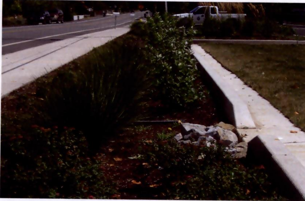
Figure 4.6. An LID swale with check dams to slow the flow of water and increase infiltration.
