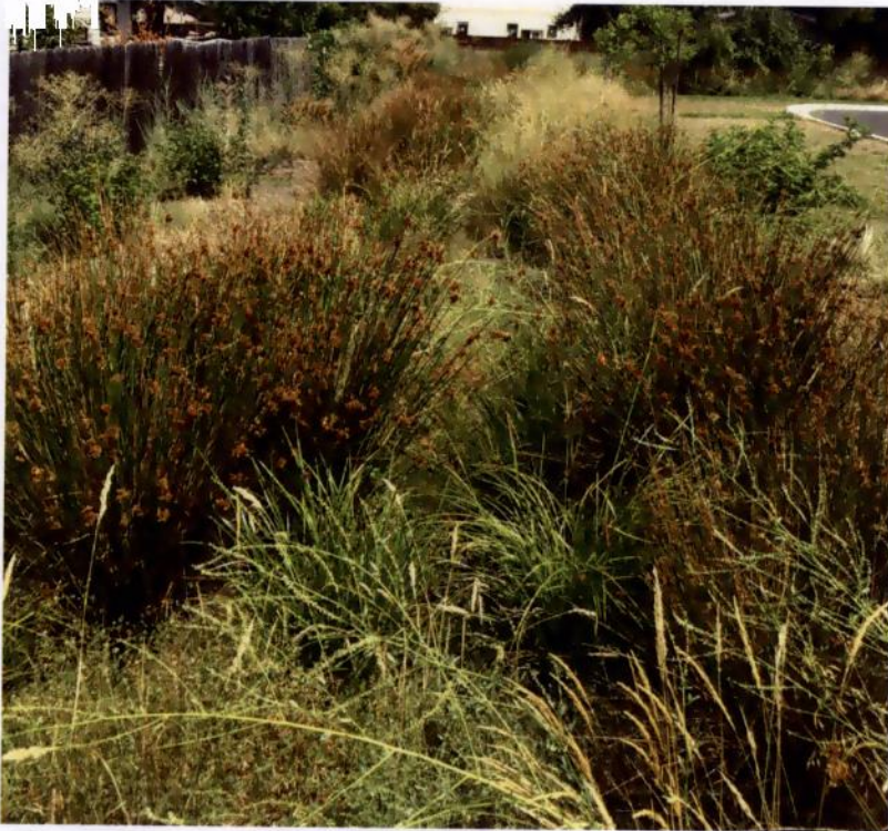
Figure 4.10. A water quality conveyance swale with dense mature vegetation that provides filtering of stormwater runoff.
