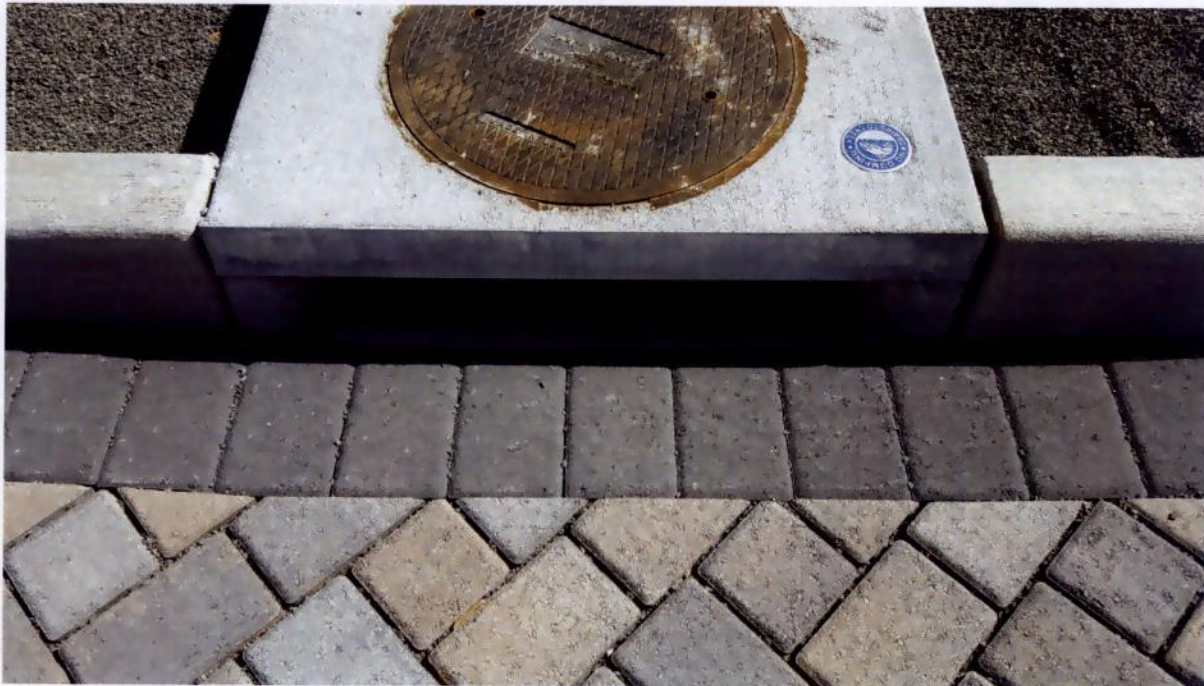
Figure 4.3. Porous pavers intercept rainfall and infiltrate it into the ground, the catch basin will only receive runoff from large storm events.
