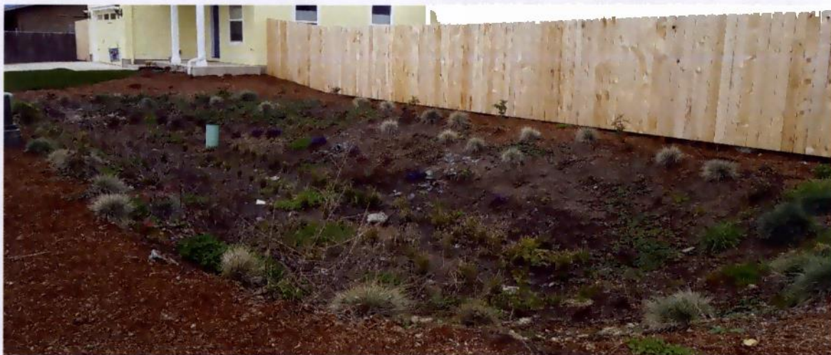
Figure 4.5. Neighborhood scale residential rain garden six months after installation.
