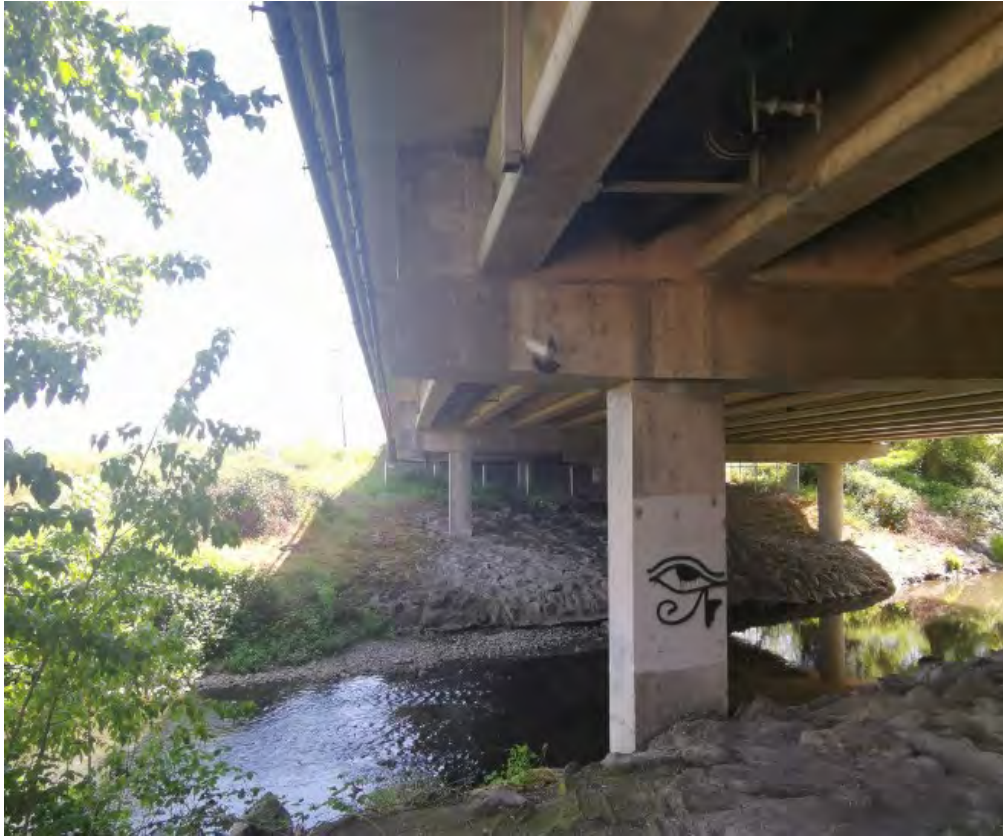
Photo 7: Pine Street Bridge and Pipe on the Beidge
