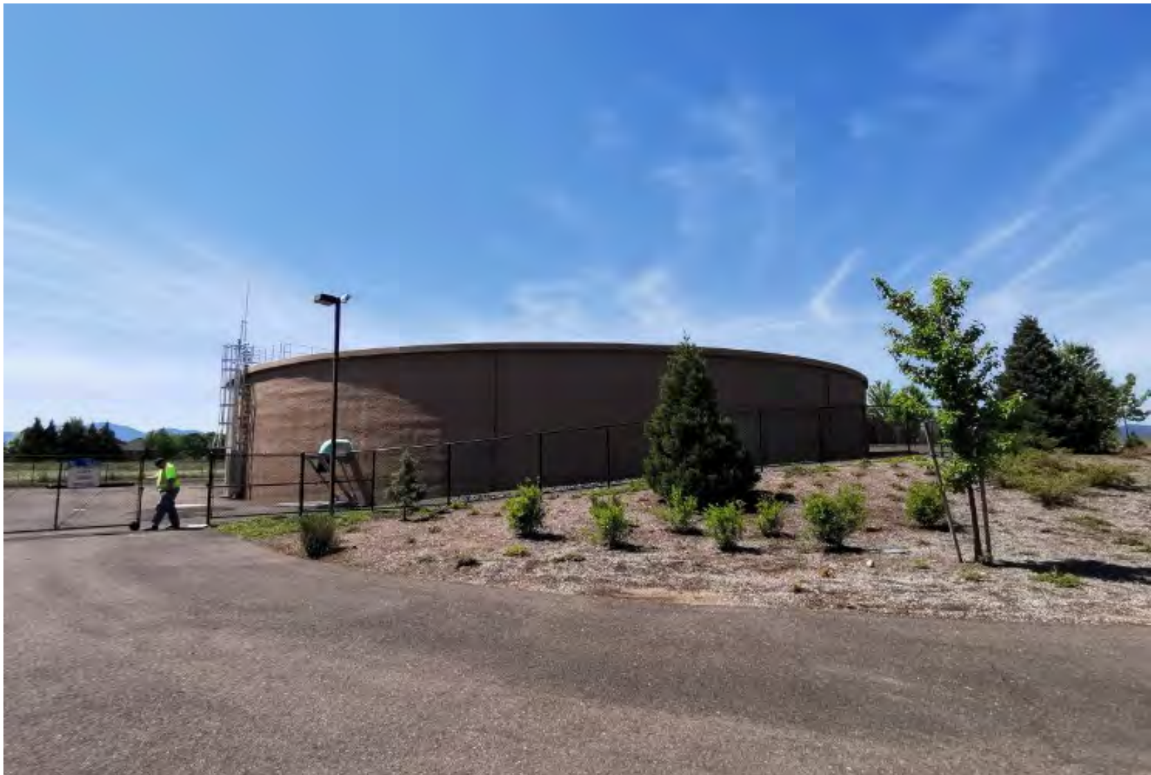
Photo 6: Vilas Reservoir (looking at the entrance and north side of reservoir)
