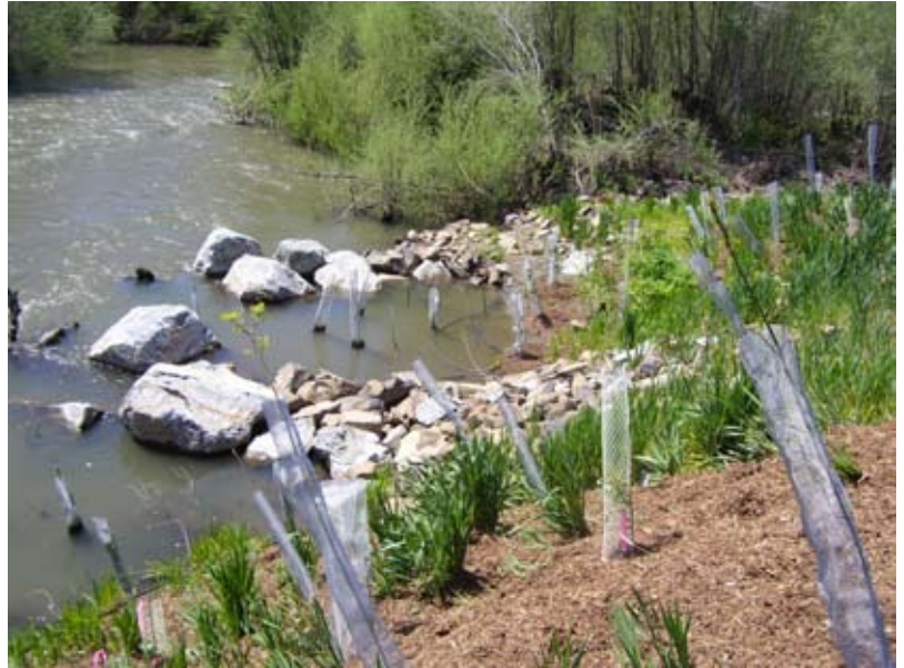
Figure 1.—A newly installed riparian planting along Bear Creek, Jackson County.
