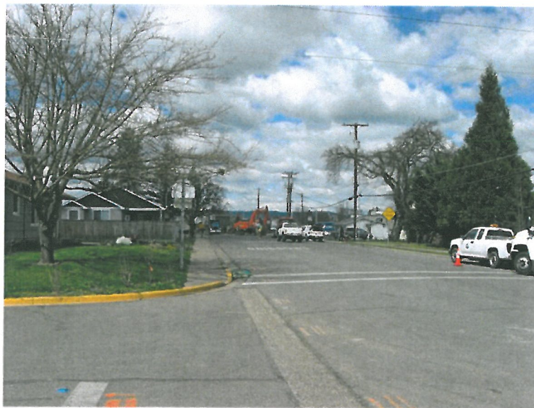
3rd Street Storm Drain Project
