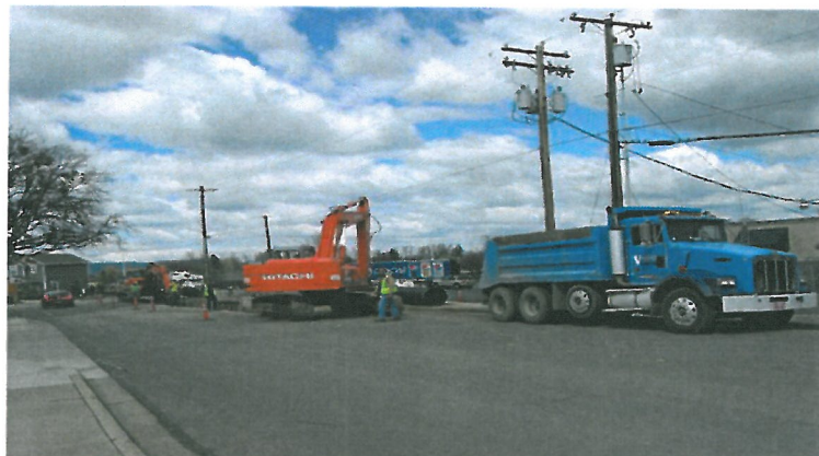
3rd Street Storm Drain Project
