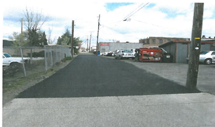
Paved alley between 2nd and 3rd
