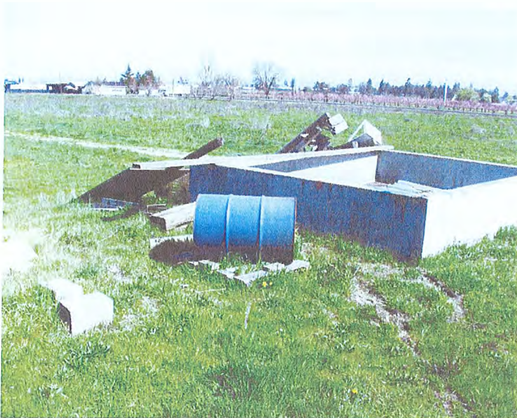
Photograph 7. A concrete containment was constructed for an aboveground storage tank used for diesel fuel. The 55-gallon drum, currently empty, previously held kerosene for a shop heater.
