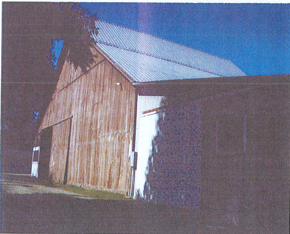
Photograph 2. View west at the large barn on the Site.
