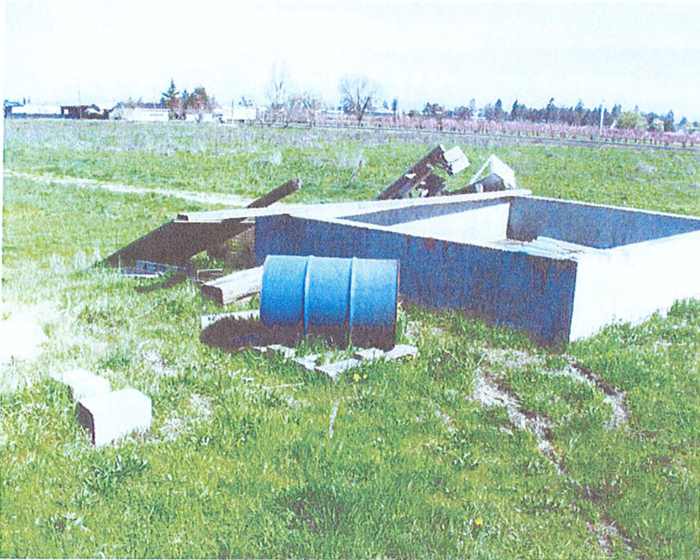
Photograph 7. A concrete containment was constructed for an aboveground storage tank used for diesel fuel. The 55-gallon drum, currently empty, previously held kerosene for a shop heater.
