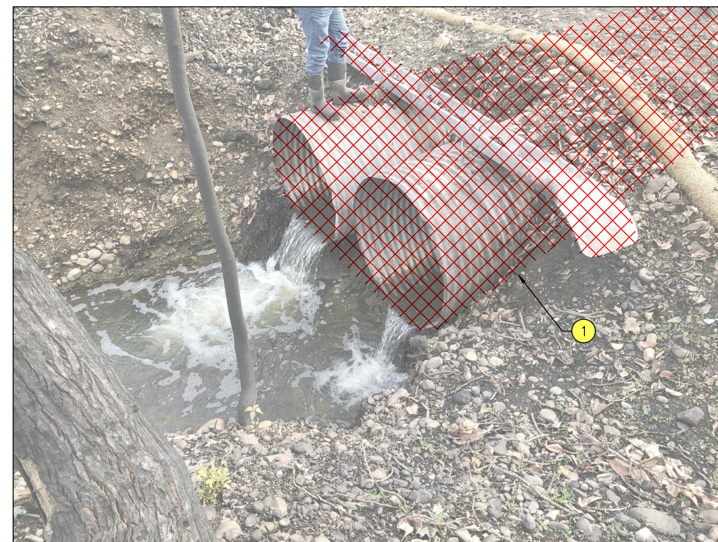
2 CULVERT OUTLET DEMOLITION NOT TO SCALE
