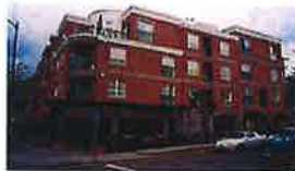
Corner retail with prominent entry.
