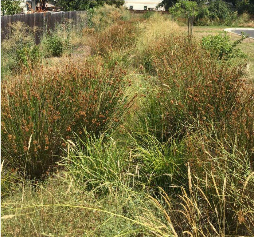
Figure 4.10. A water quality conveyance swale with dense mature vegetation that provides filtering of stormwater runoff.
