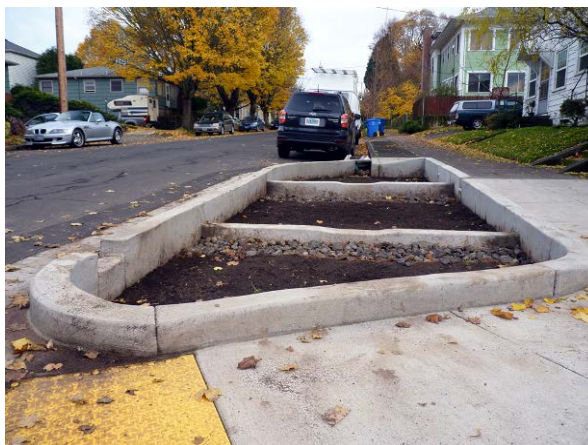
Figure 4.7. A residential above-ground stormwater planter (left). An in-ground stormwater planter with concrete check dams in a public street before planting (right). The centerline (looking straight up the center of this photo) slopes at less than 1%. Concrete check dams were needed because the street slopes more than 1%. Grades parallel to the check dam are flat.
