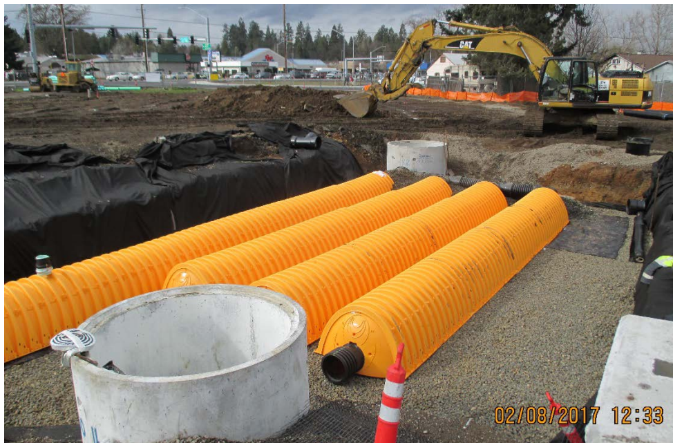
Figure 4.11. Stormtech Chambers are one example of a stormwater treatment technology that has been pre-approved by the Rogue Valley Stormwater Advisory Team.
