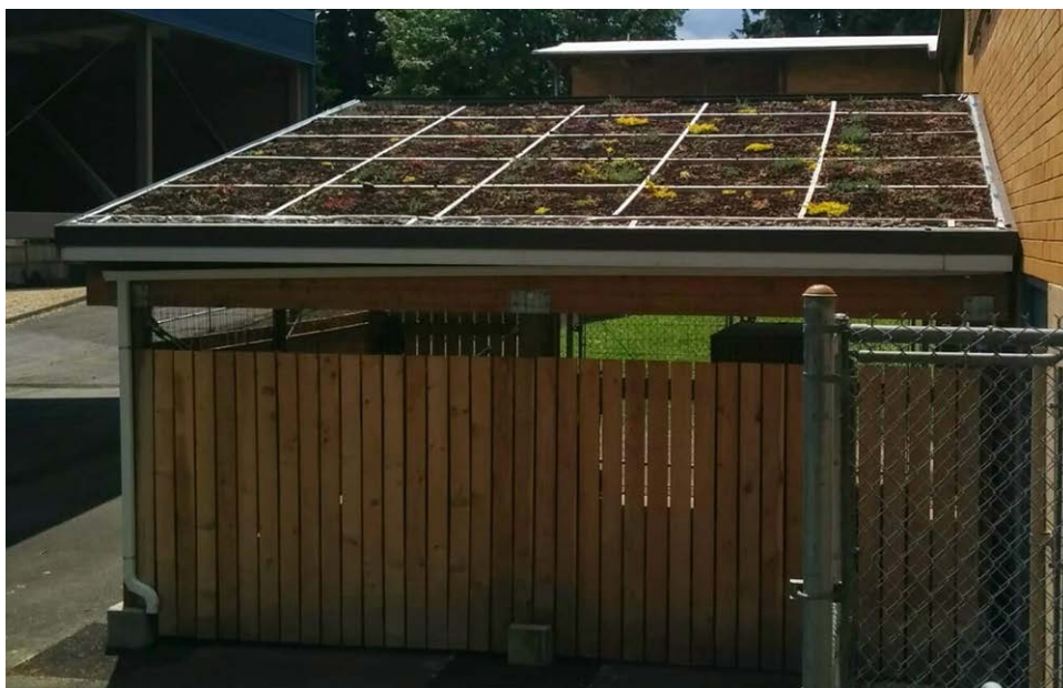
Figure 4.1. Growing medium on this small vegetated roof was stabilized with lumber to keep it from sliding down the steep slope.
