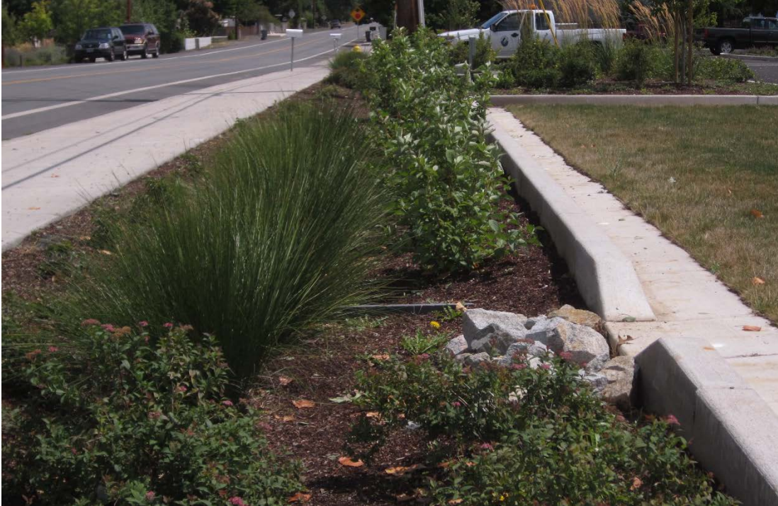
Figure 4.6. An LID swale with check dams to slow the flow of water and increase infiltration.
