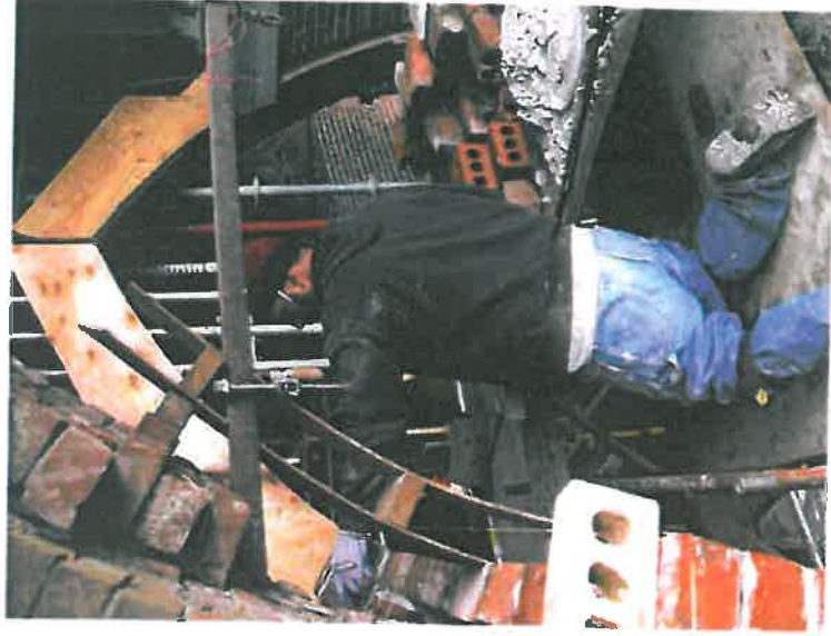
Restoring the historic arch in Lake Oswego's Iron Works.
