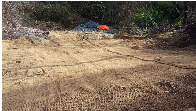
Jute matting protecting an excavated slope on a 1200-CN permitted project.
